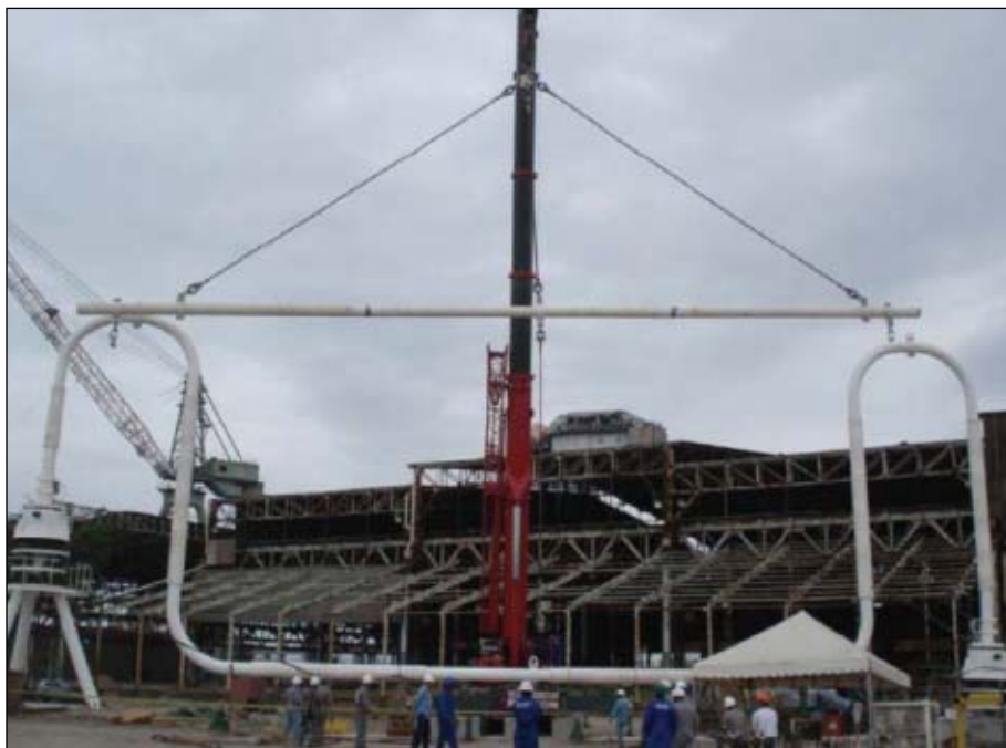
The rigid-base jumper's (RBJ) pipe measures 18 in. OD and 1.125 in. WT. Cyclic loads from thermal expansion caused by shutdown and offtake spool motions must also be assessed to gauge RBJ fatigue damage (Fig. 2).
